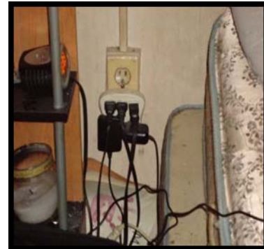
Unsafe Wiring
