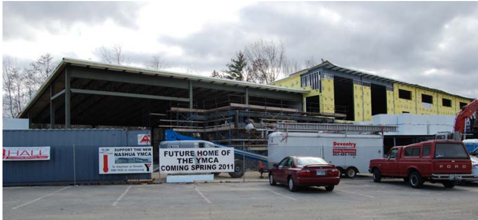
New YMCA on Stadium Drive – Est. Completion Spring 2011
