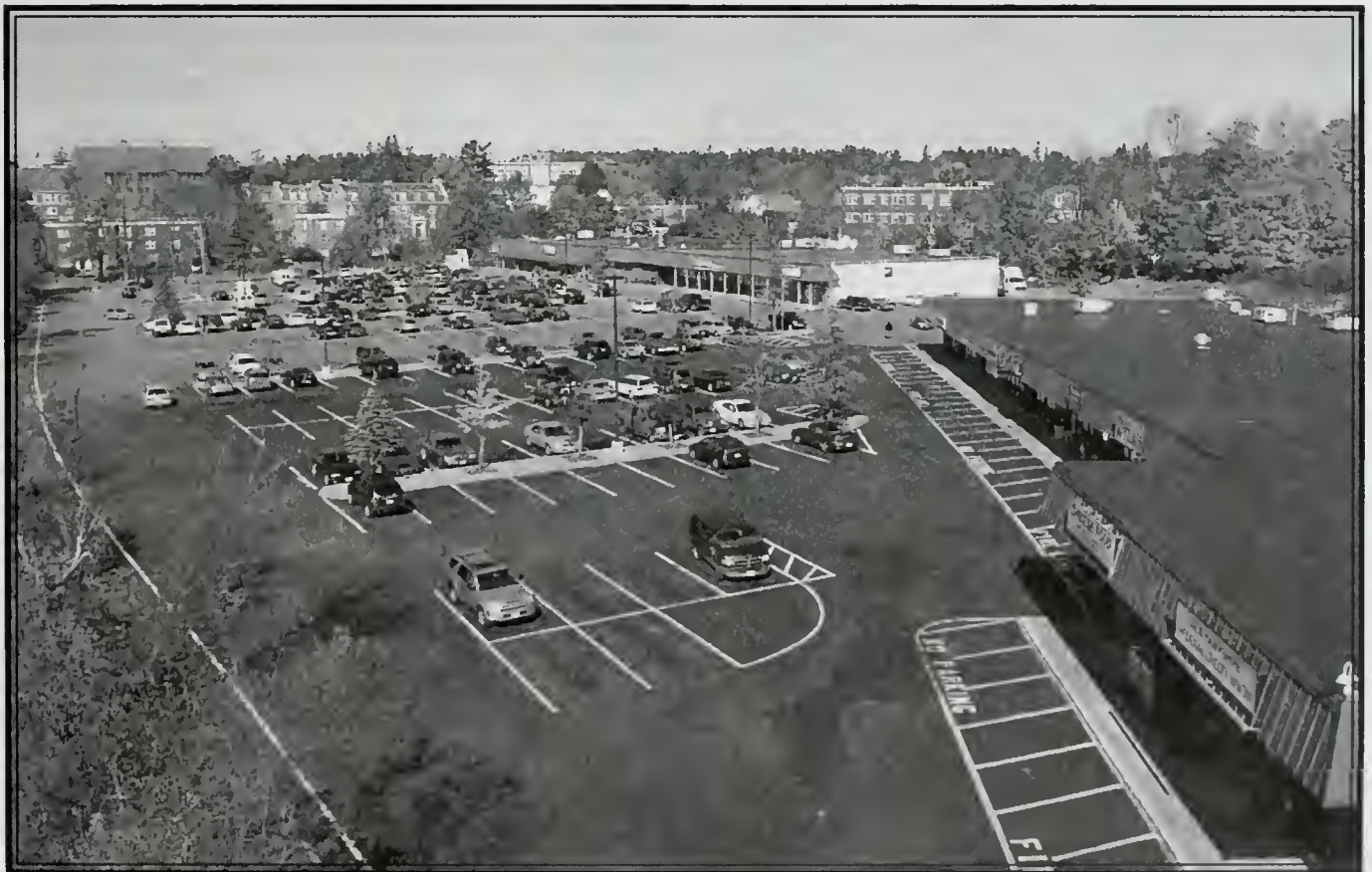
The existing Mill Pond Plaza. PHOTO COURTESY FRANCOISE MEISSNER, CONDOR AERIAL IMAGE SYSTEM
