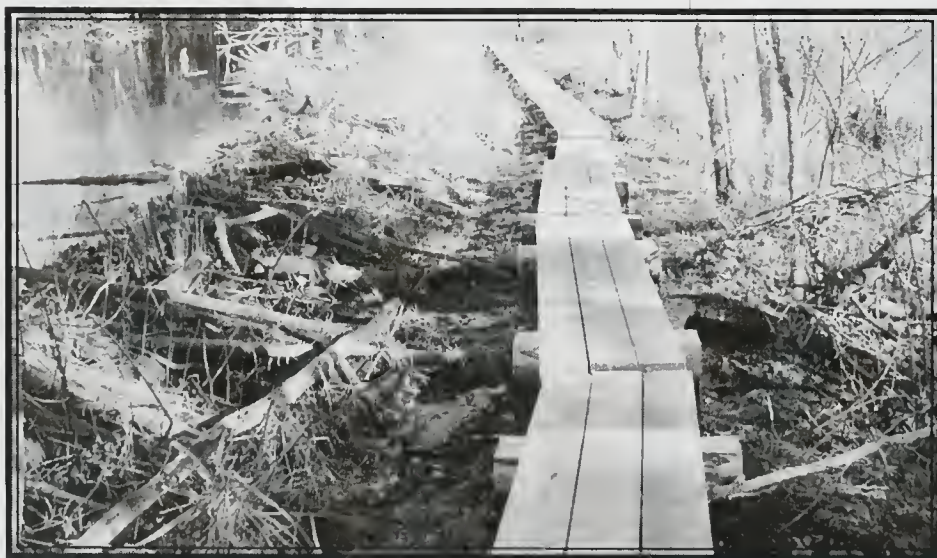
Looking East at the westernmost bridge on Longmarsh Trail. The beaver dam is to the left of the walkway. This bridge is very long and not all of the western end and the eastern end are visible in the photo. PHOTO BY FRANK L. PILAR
