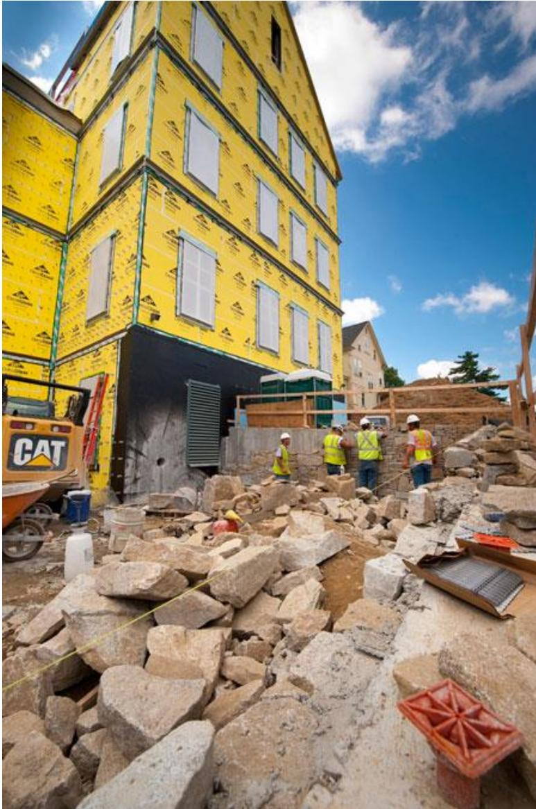
The project is the result of painstaking work by Stoneage Stoneworks of Berwick, Me., and it is one of the first finished exterior aspects of the new business school now under construction. The stone wall serves as a veneer that covers drab concrete retaining walls, but it also draws the eyes of passersby to the building's upper stories -- while looking very much like the sturdy foundation of an old New Hampshire mill or barn.
