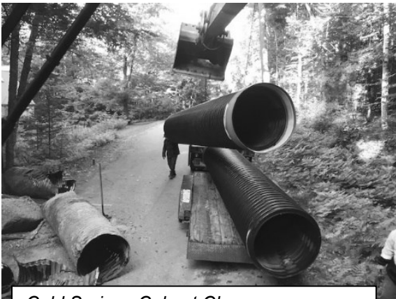
Cold Springs Culvert Change
