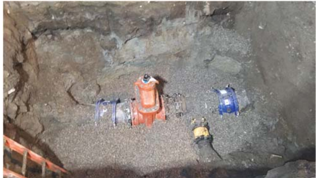
New water 14" gate installed
