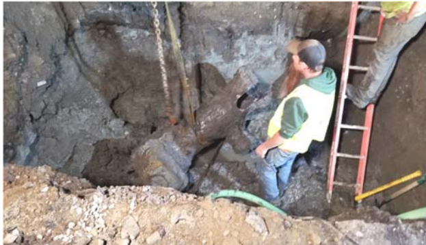
Removal of the old 14" water gate
