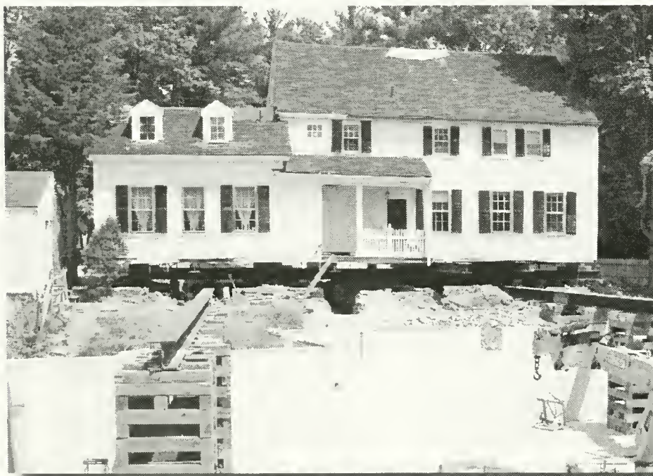
The foundation is poured and the platforms are in place to begin moving the Dewey Hannah House located on Packers Falls Road. RICHARD LORD PHOTO
