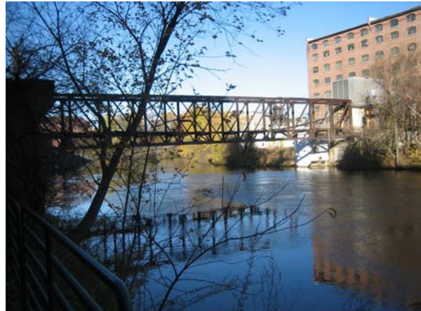
Cotton Transfer Bridge (aka Pratt Truss Bridge)
