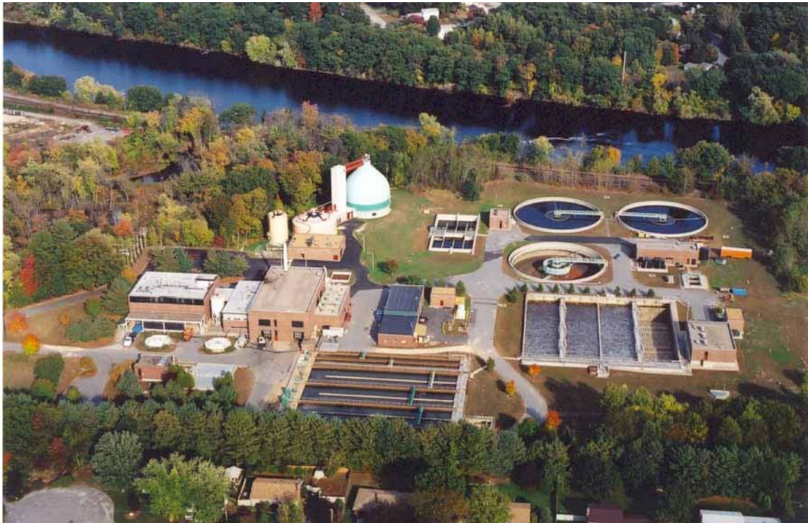
Aerial view, Wastewater Treatment Plant
