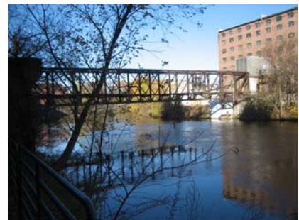
Cotton Transfer Bridge (aka Pratt Truss Bridge)
