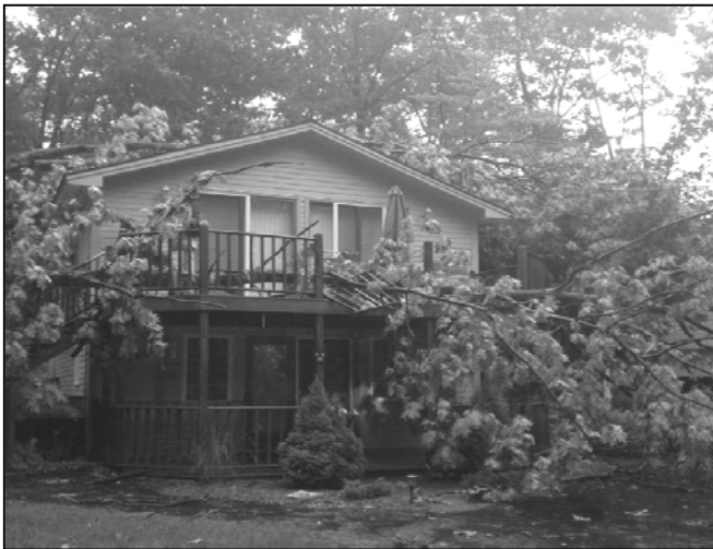
Storm Damage – Dockham Shore Road
