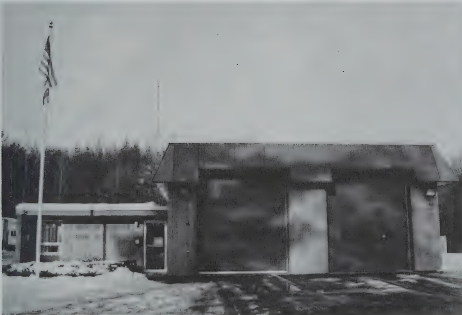
SOUTH END FIRE STATION DURHAM ROAD BUILT 1967
