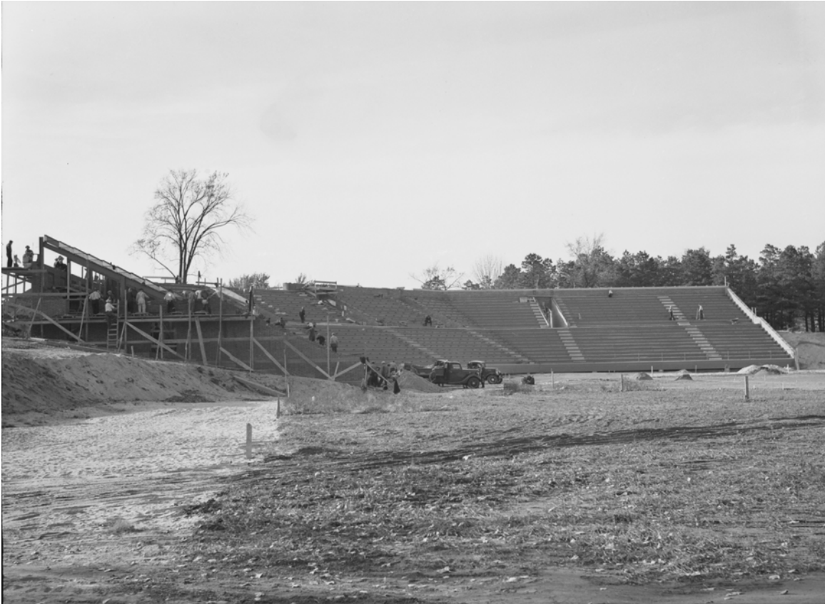
Municipal Stadium being built by WPA, Nashua, NH (Holman Stadium) National Archives Call Number 068-N-5295-A: Athletic Fields, WLH 10/1936
