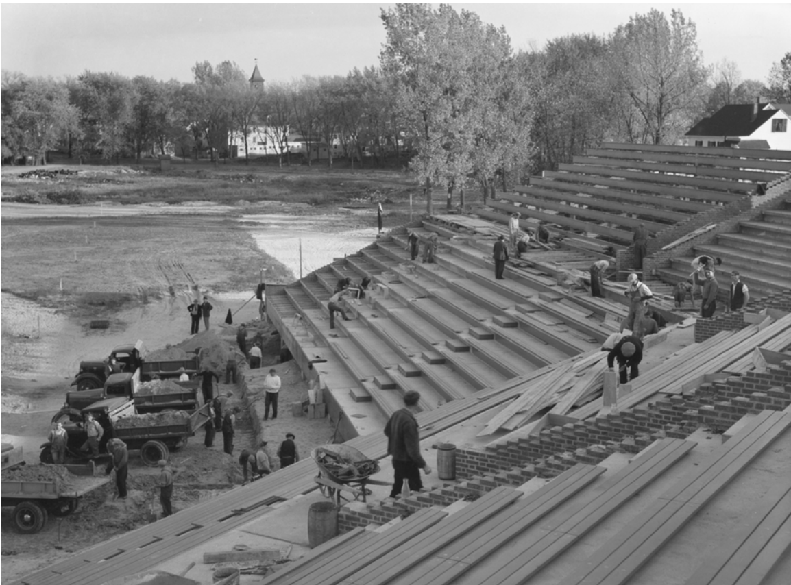
Holman Stadium Construction – 1936
