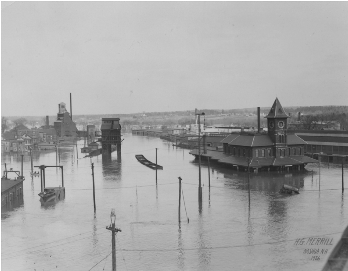
(J.F. McElwain) roof. Johns Mansville Co. at right. Slight ripples just front of depot (left) are five automobiles just covered with water. 1936 flood. Donor: Helen L. Kimball, Milford, 4/1/1987. Photo Courtesy of Nashua Public Library.
