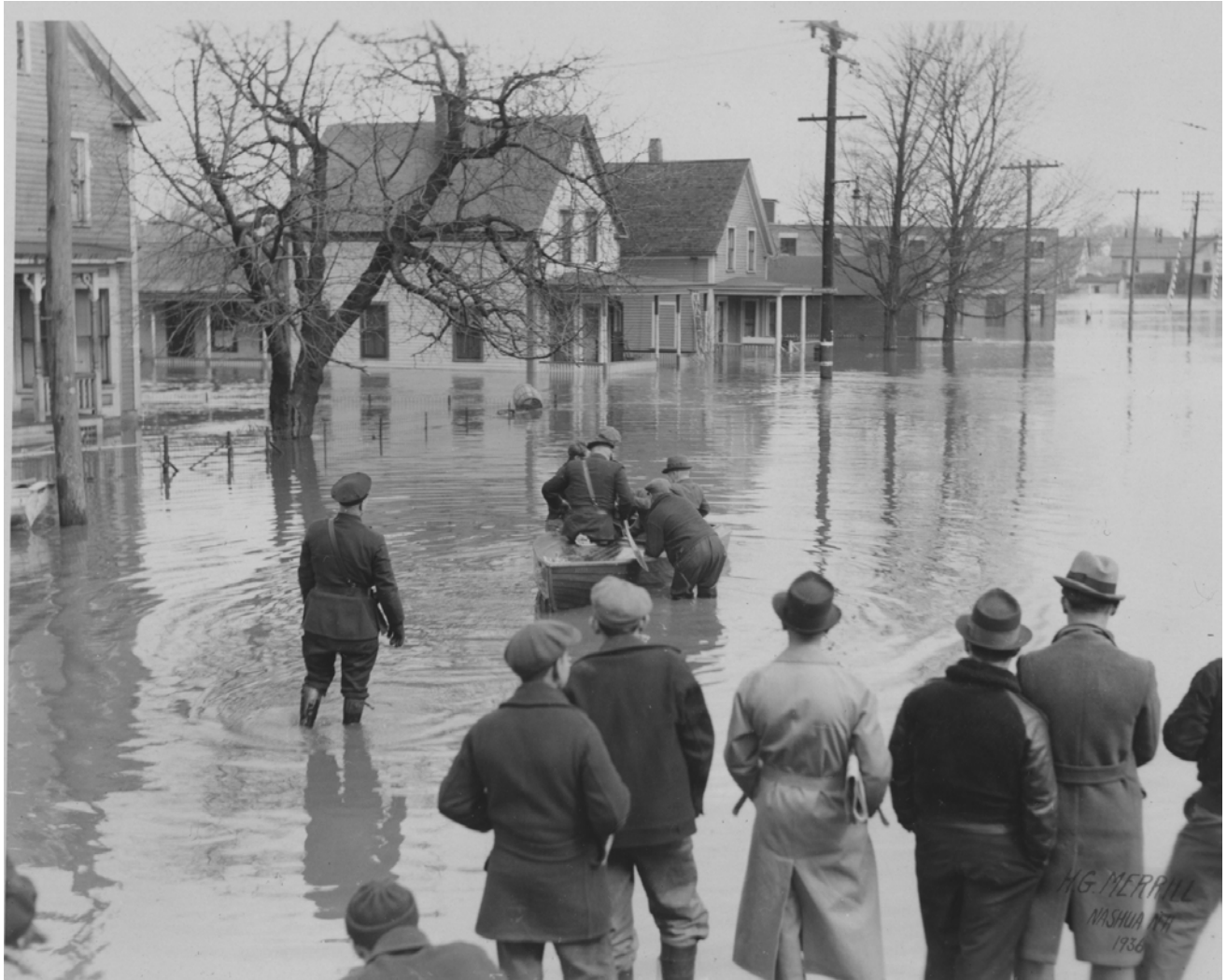
Chief Goodwin and officers getting power boat running to bring refugees from houses on Crown Street. Photo courtesy of Nashua Public Library
