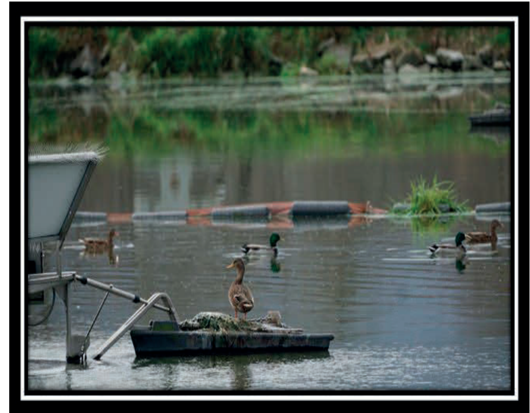
ON DUTY COLEBROOK WASTEWATER TREATMENT FACILITY Photo Courtesy Susan Zizza
