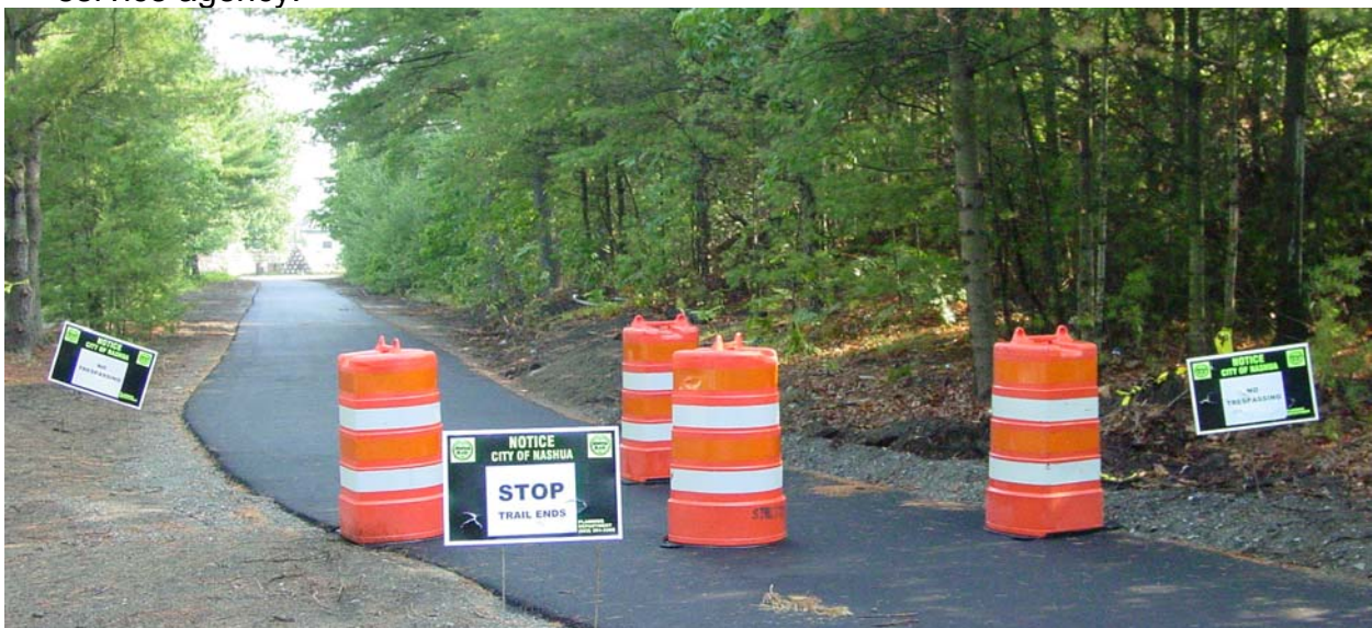
Paving of Nashua River Trail
