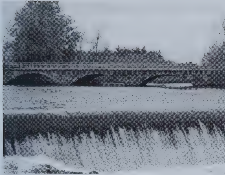
North Main Street Bridge
