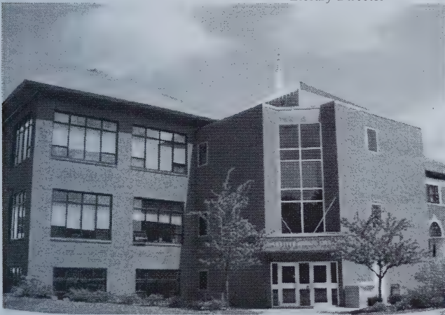
Rochester Public Library Addition
