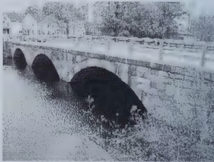
North Main Street Bridge
