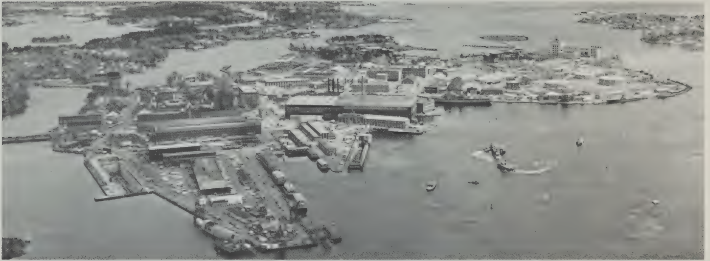
Aerial view of U. S. Naval Activities, Seavey Island. Portsmouth Naval Shipyard employs over 8,000 who devote their full-time effort to the construction, conversion, and overhaul of the Navy's submarine fleet. (Left background, Kittery Point; center background, Gerrish Island; right background, New Castle)
