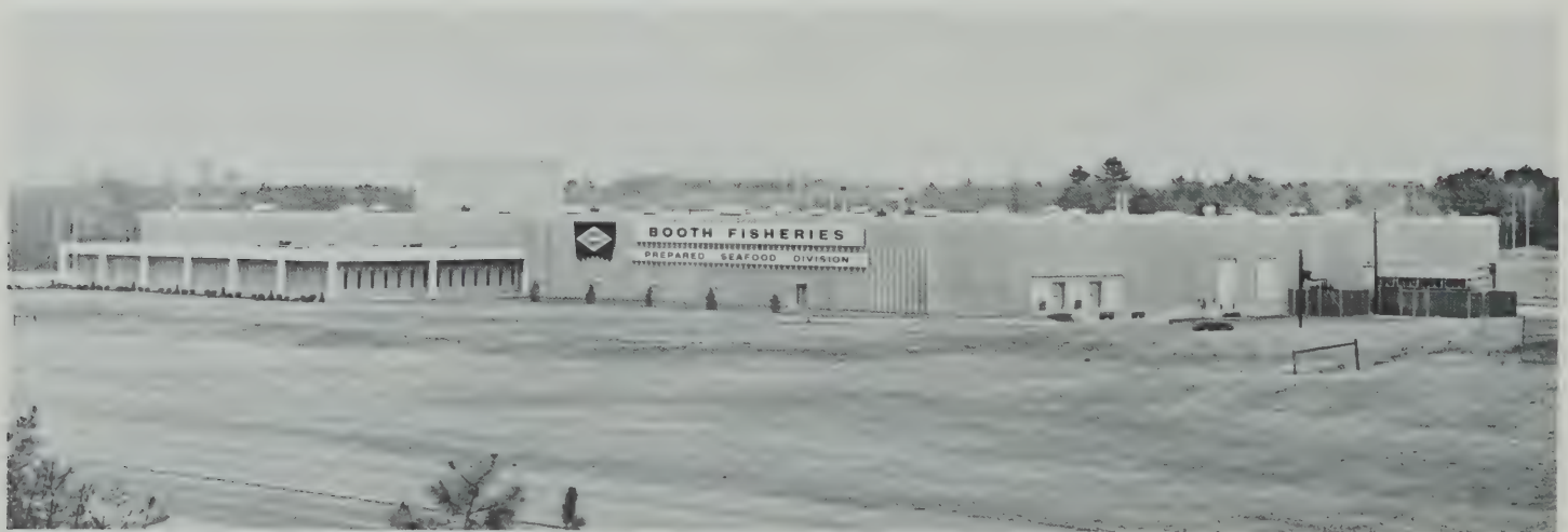
This 148,000 square foot plant of Booth Fisheries is located at the Federal and Interstate cross-roads of the New Hampshire Seacoast region. A $4.5 million plant, it is the largest and most modern in the prepared seafoods industry.
