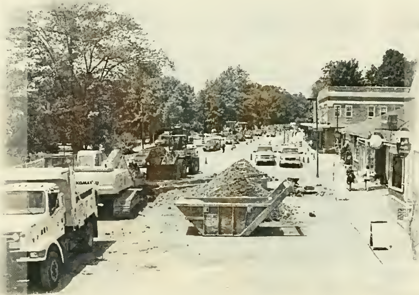
Main Street under construction
