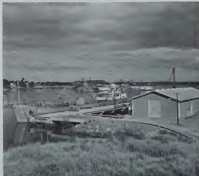
State Port Terminal Wharf
