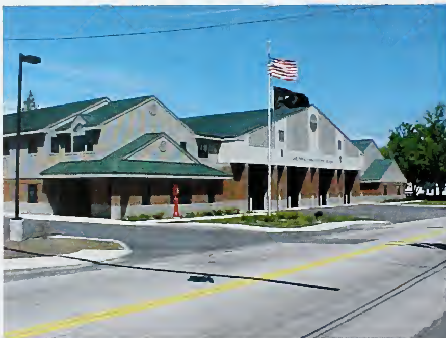
Lake Street Community Fire Station – Nashua Fire Rescue Headquarters photo by Roger Hatfield, Asst. Fire Chief
