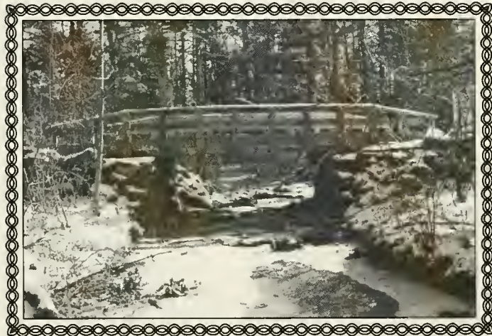
TOP: As part of the College Brook Project, the once narrow pedestrian bridge, located off Mill Pond Road, was widened. BOTTOM: Residents of the Mill Pond road area were pleased when the long awaited College Brook bridge installation was completed in October.
