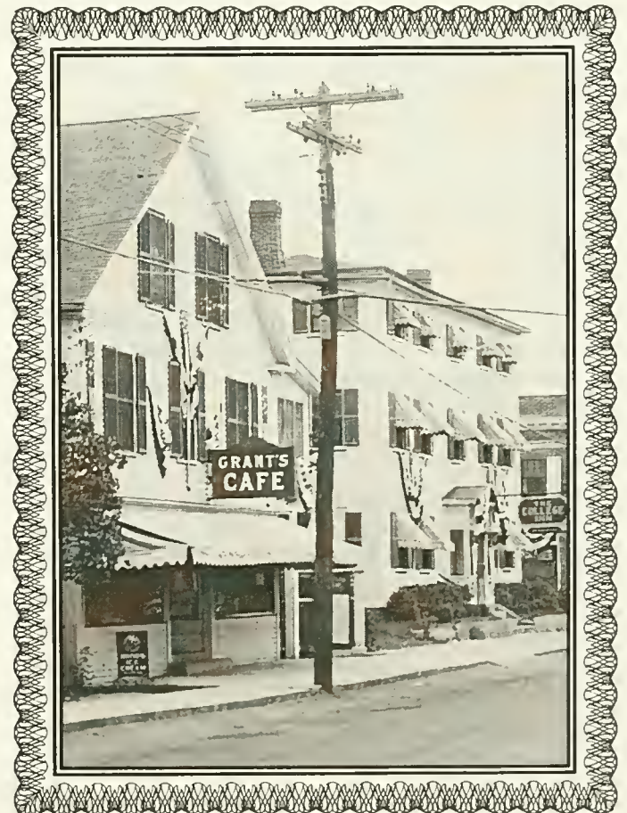
1932 at Durham's Main Street and Mill Road Intersection showing Grant's Cafe and the College Inn. PHOTO COURTESY OF THE DURHAM HISTORIC ASSOCIATION MUSEUM
