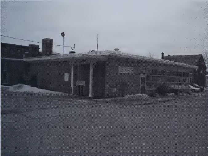
Rochester Revenue Building
