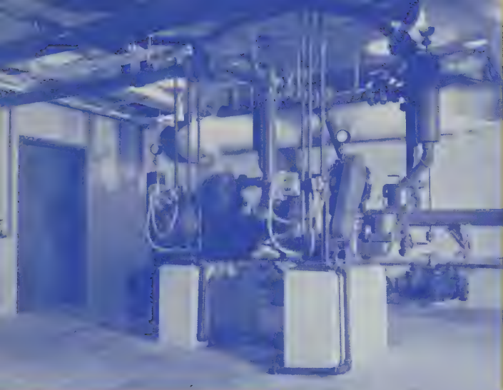
Sludge Pumps — Lower Level
