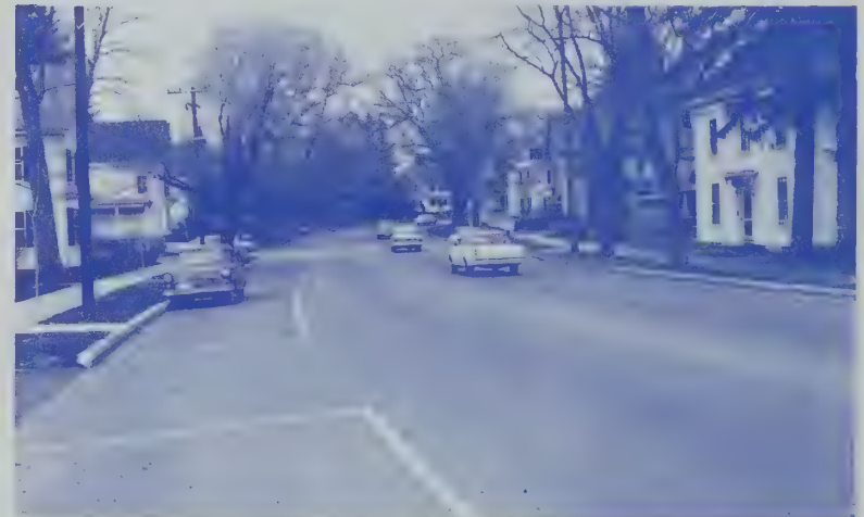
Improved Middle Street Section
