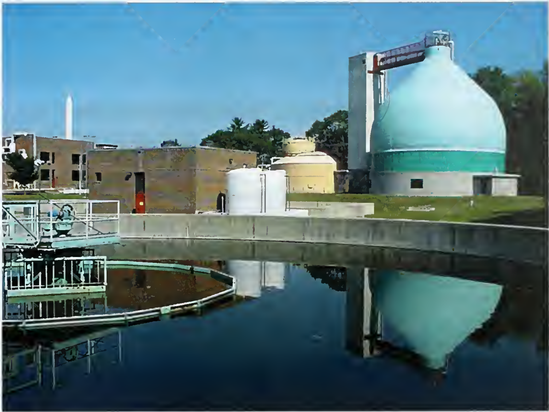
New Anaerobic Digester, dedicated in May 2001, was fully operational by summer.
