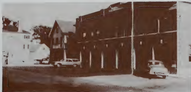
New apron front of Fire Station.
