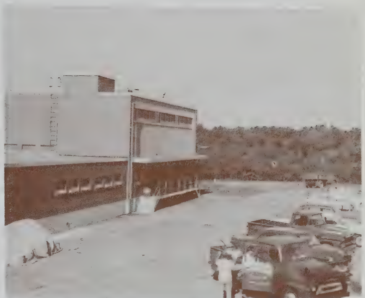
Water treatment plant, Madbury, New Hampshire.
