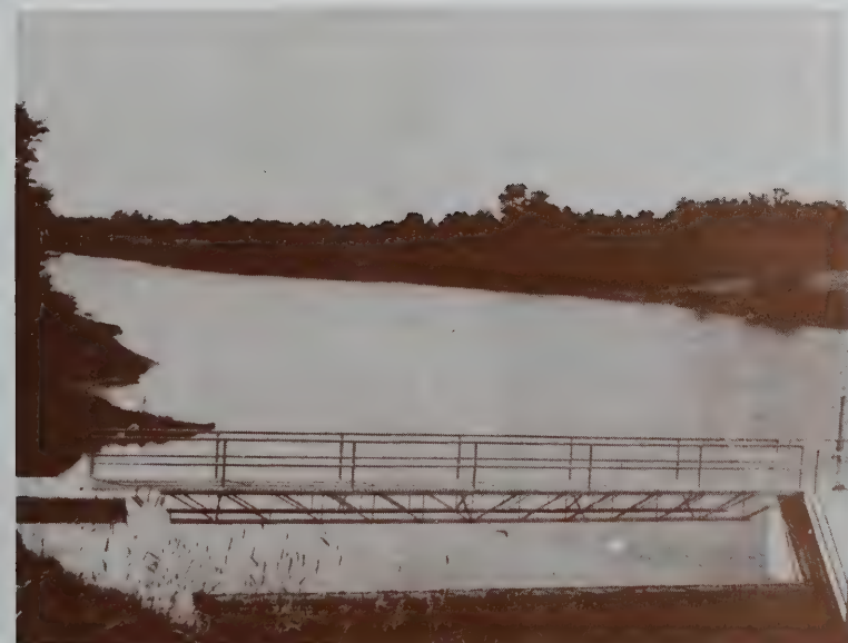
Spillway — Bellamy Dam.
