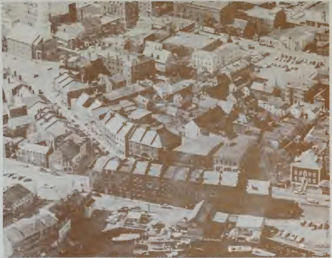
Aerial View High/Hanover Street Area (before Parking Area Construction).
