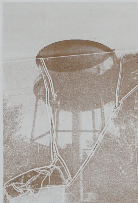
Elevated Water Tank — Wentworth Acres. Capacity of storage 200,000 gallons.
