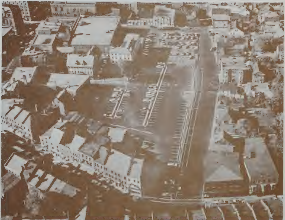
Aerial View High/Hanover Street Parking Area.
