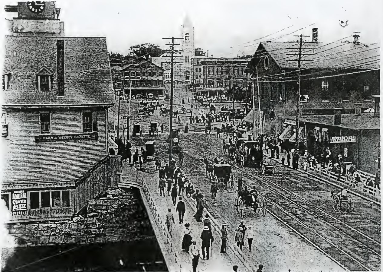
Main Street, looking north toward Railroad Square
