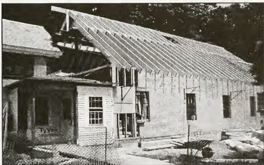
Roof trusses are almost all in place.
