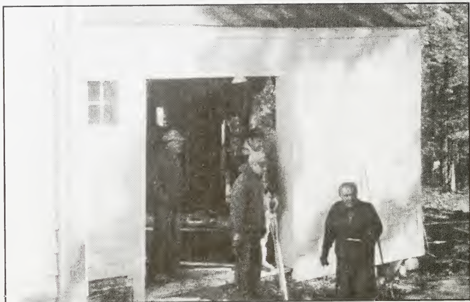
Getting ready to begin demolition of the barn.
