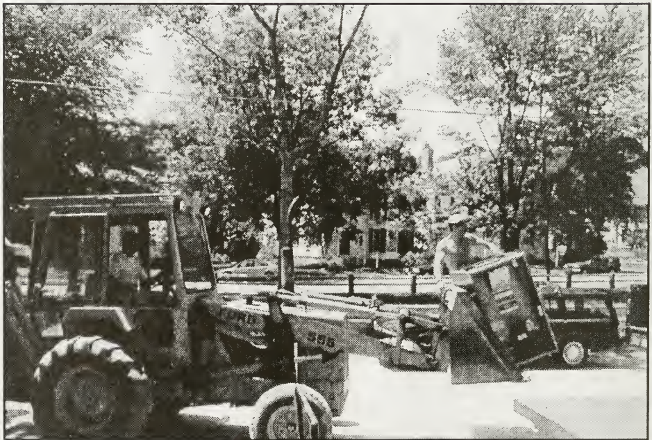
Highway personnel working on the sprinkler project
