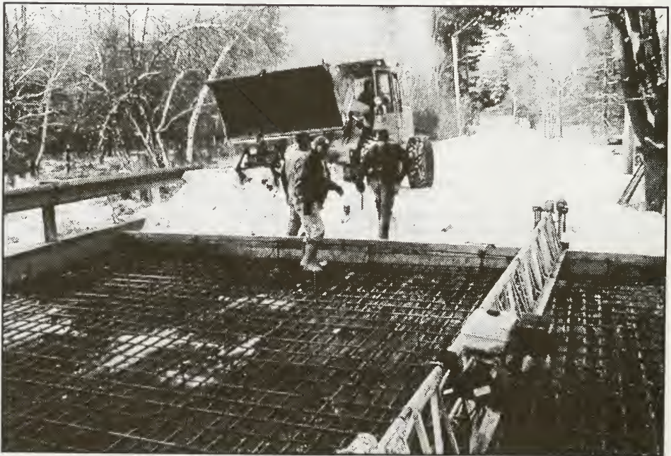
Bridge repairs on Templeton Turnpike over Priest Brook
