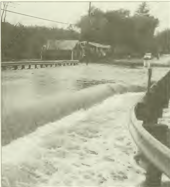
Washout at Hamel Brook on Newmarket Road, October 1996. (photo courtesy Michael D. Golding)
