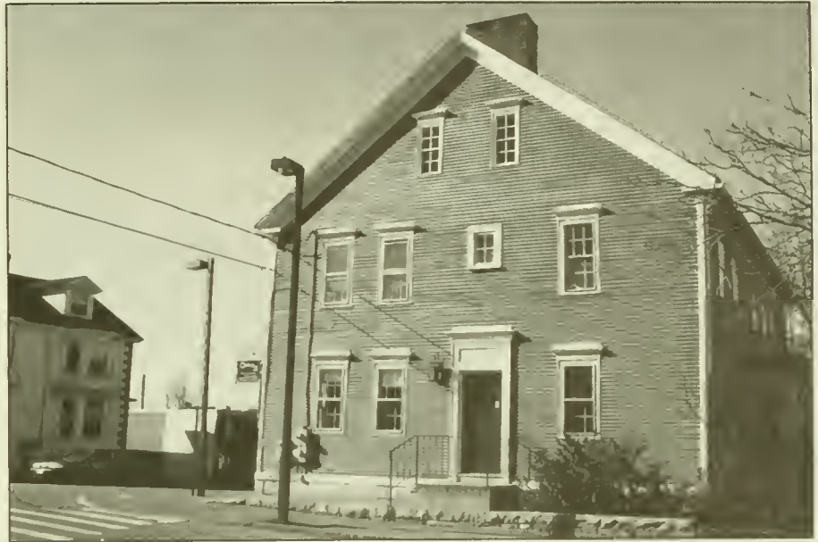
Joshua Ballard House, C. 1790, restored east wall.
