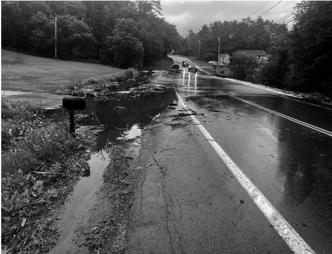
Flooding on Jefferson Road Photo by Stanley Holz
