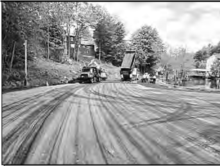
Photograph of River Road shimmed and resurfaced with 1.5" of new asphalt.
