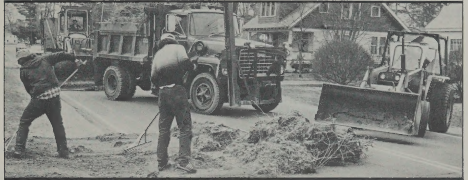
Fall clean-up at South Street and Jordan Avenue. (Concord Monitor photo)
