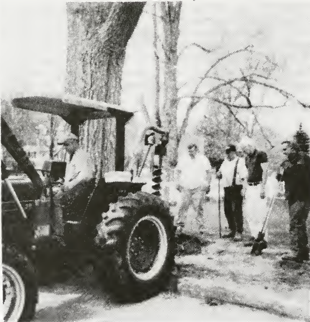
Construction of the new Library Fence
