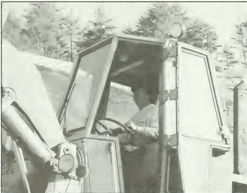
Michael Douglas screening sand at Packers Falls gravel pit.
