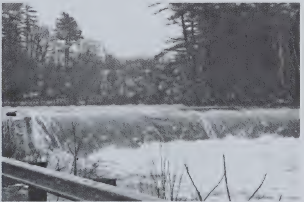
Water rages over the dam on Antrim Road near Alberto's Restaurant
