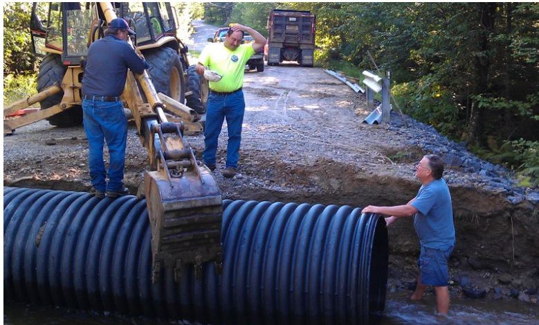
Bringing back the washed out culvert on Long Pond Road
