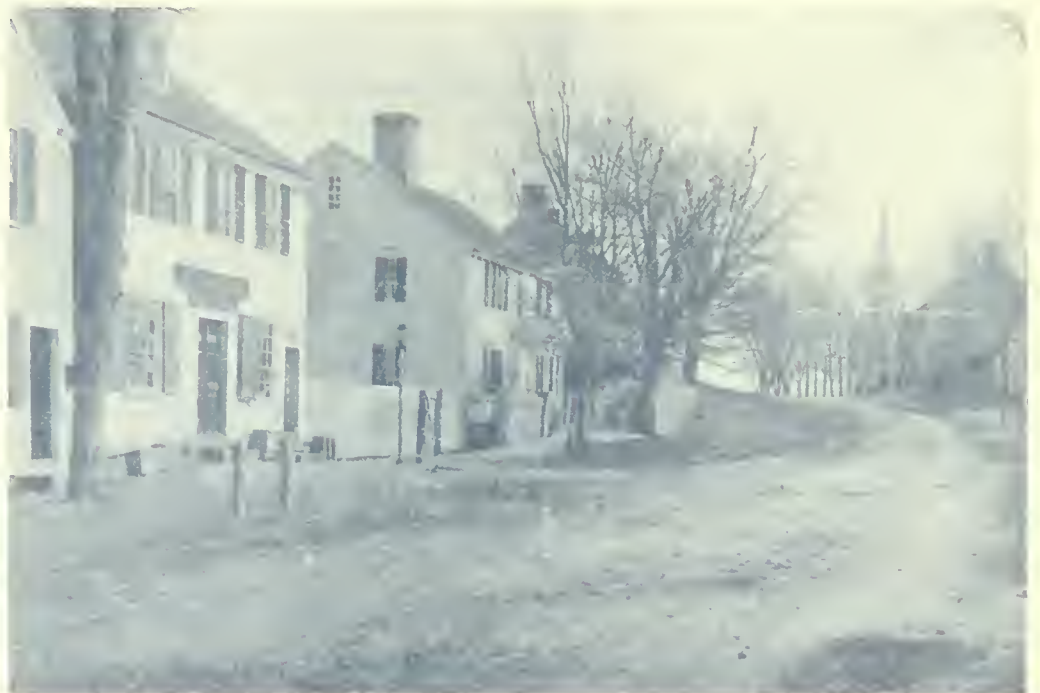
Looking up Main Street towards the Community Church in the 1890s.
