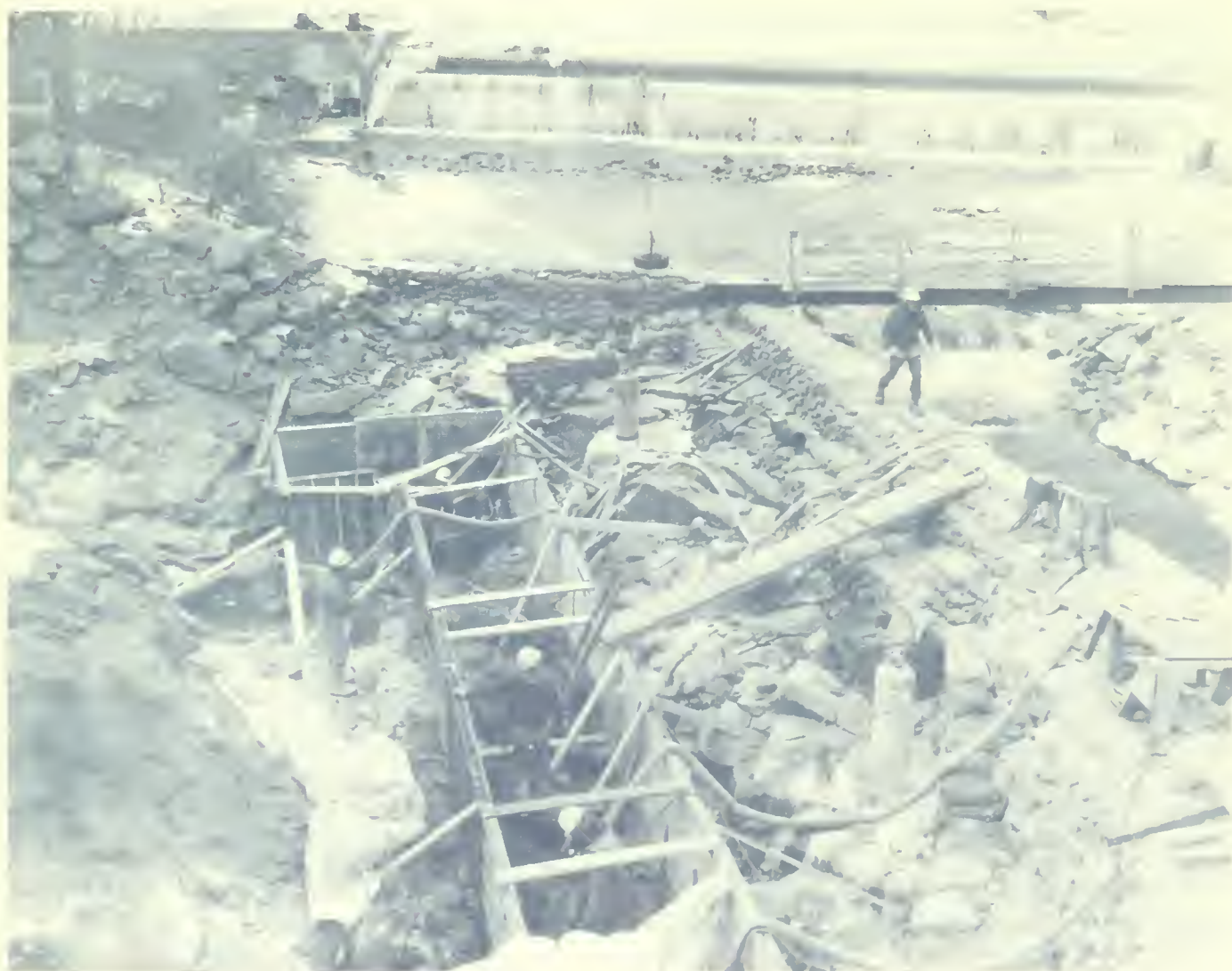
The construction of the new Oyster River Bridge
