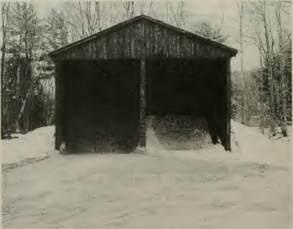
Highway Department Sand/Salt Shed
