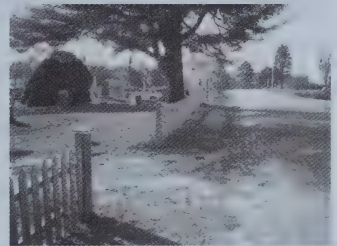
Finished picket fence and gate
