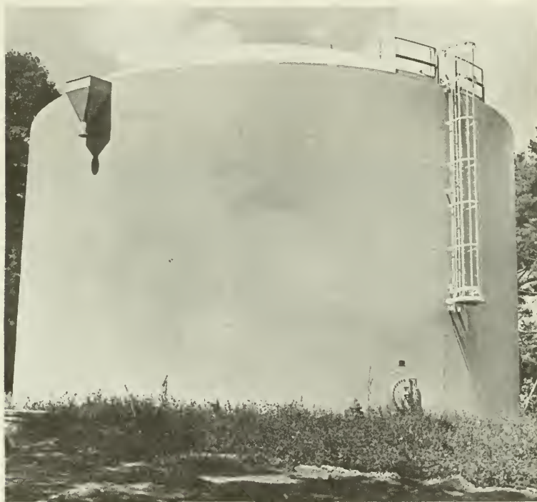
Water Storage tank on Beech Hill Road.
