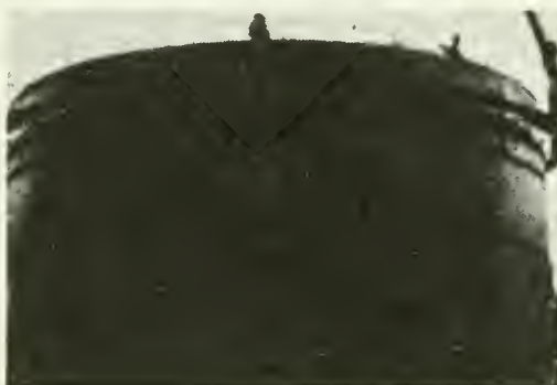
NEW 600,000 GALLON WATER TANK UNDER CONSTRUCTION
