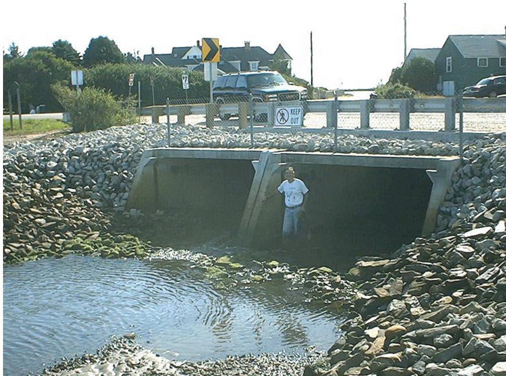
Figure 1. Old and New Culverts: upper photograph shows outlet (Gulf of Maine side) of the original 1.2 m (48-inch) culvert; pictured below is the marsh side of the new culvert (two side-by-side 1.8 by 3.6 m or 6 by 12 foot culverts).
