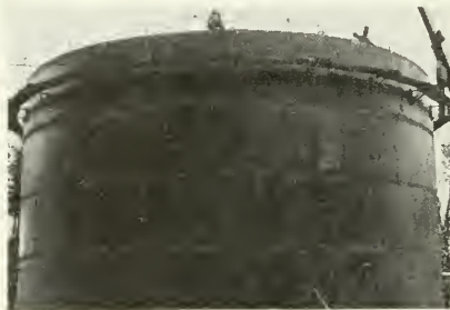
NEW 600,000 GALLON WATER TANK UNDER CONSTRUCTION
