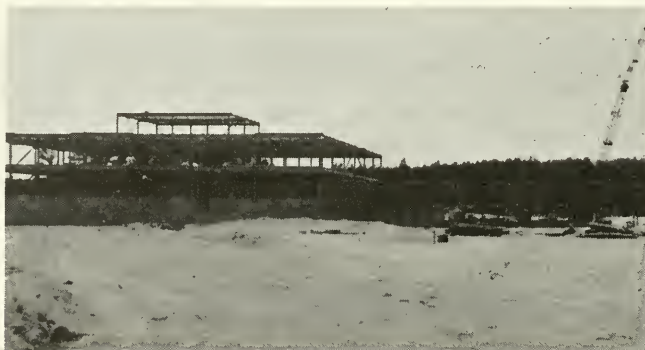
DATA GENERAL FACILITY UNDER CONSTRUCTION
