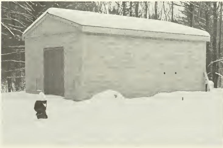
NEW WELL HOUSE IN LEE UNDER CONSTRUCTION
