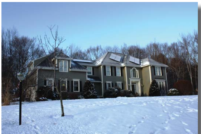
Then the photovoltaic panels were installed on top of the roof.
