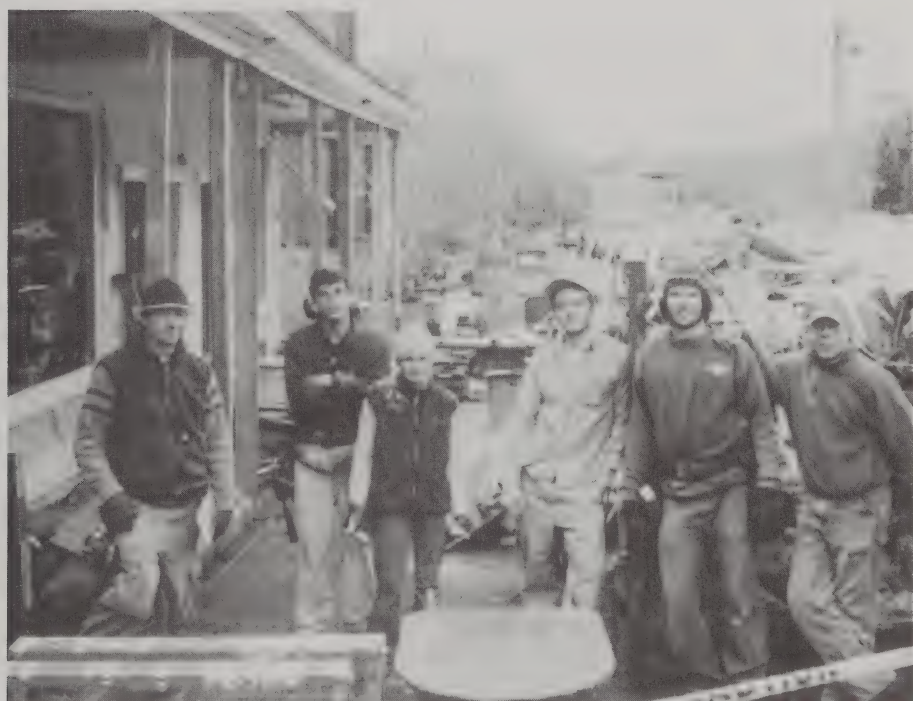
David Pickman (r) & crew restore facade of a planned antique complex.
