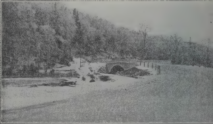
THE NEW CEMENT BRIDGE
