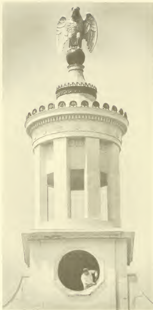
CLOCK TOWER REPAIRS
