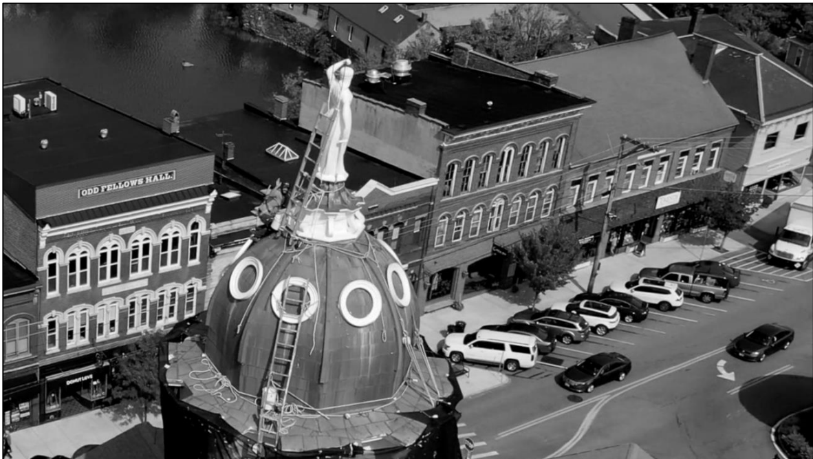
Exeter Town Hall repairs by Limerick Steeplejacks, Inc. Photo by Morning Star Aerial LLC.
