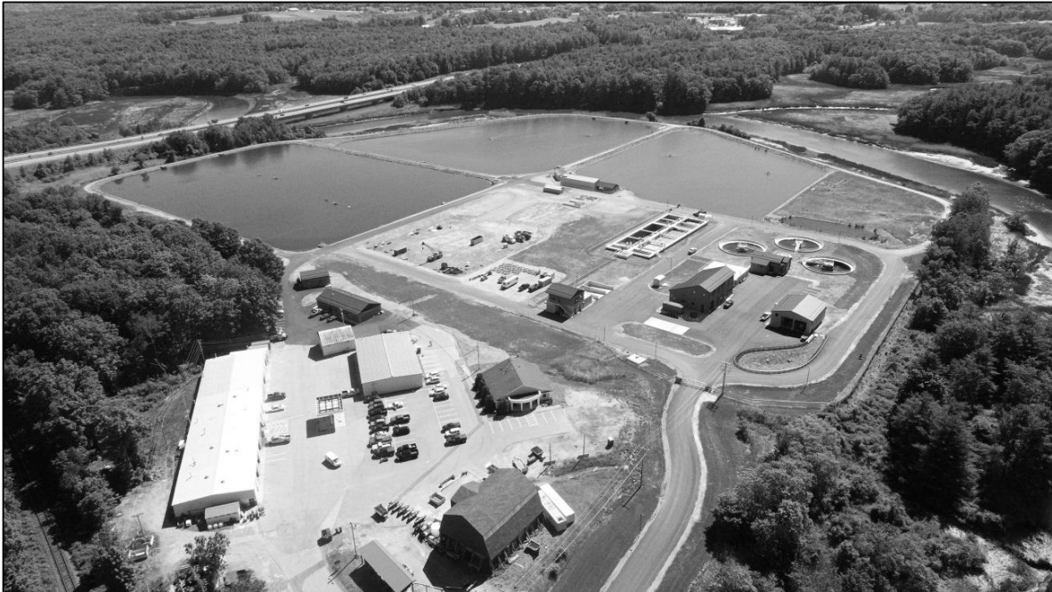
Exeter Public Works campus with upgraded wastewater treatment facility. Photo by Wright-Pierce Engineers.
