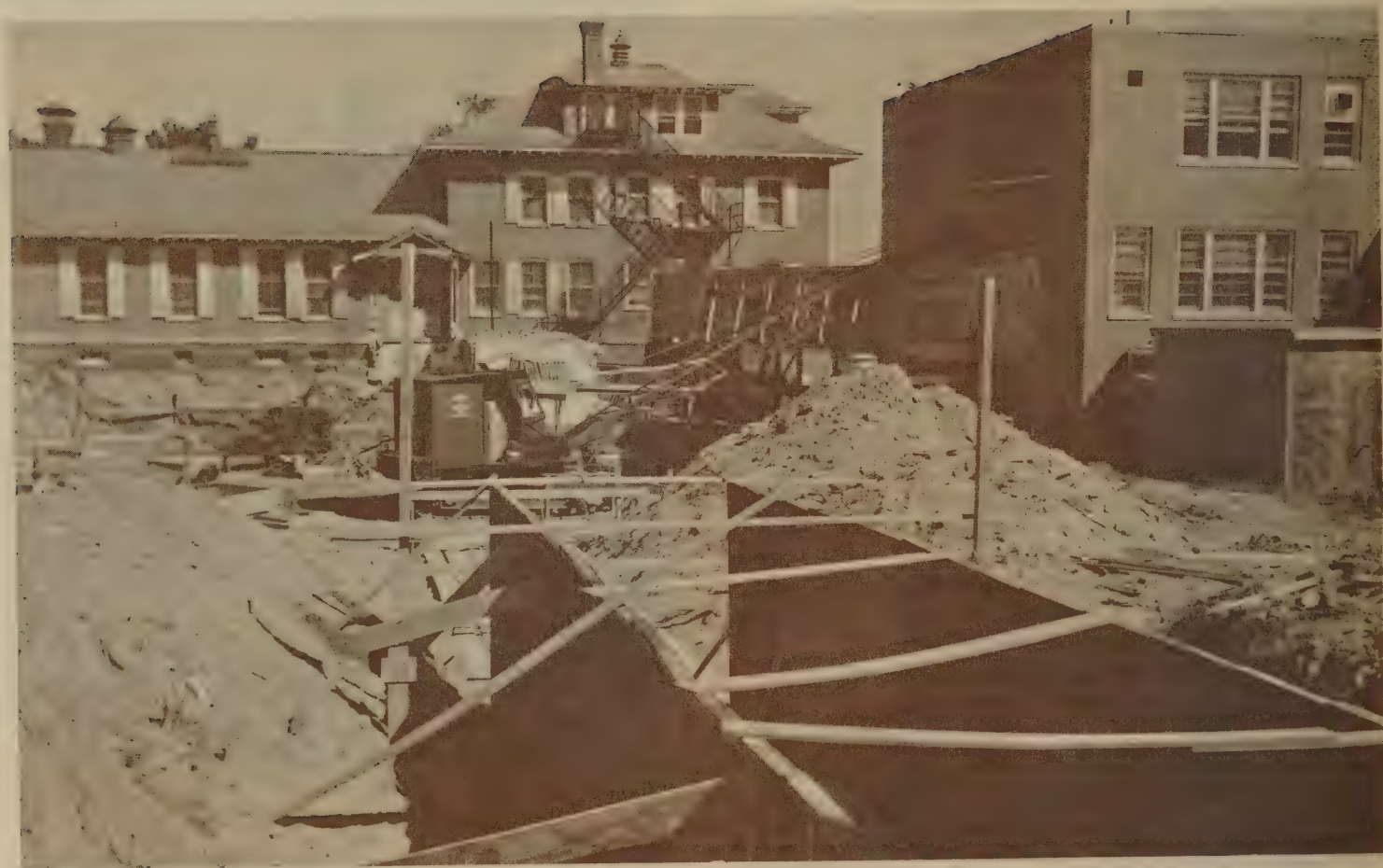
DOUGLASS ADDITION TO THE WENTWORTH-DOVER CITY HOSPITAL UNDER CONSTRUCTION
