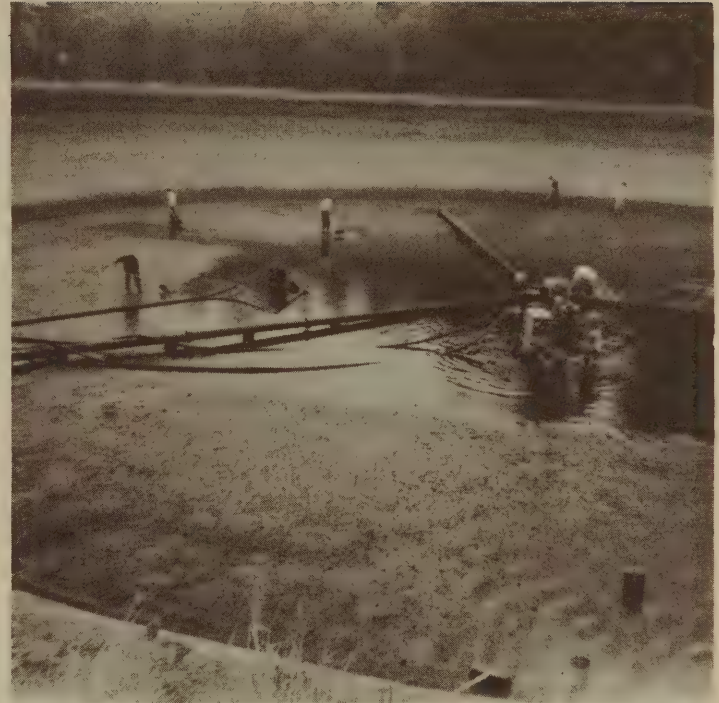
CLEANING THE RESERVOIR
