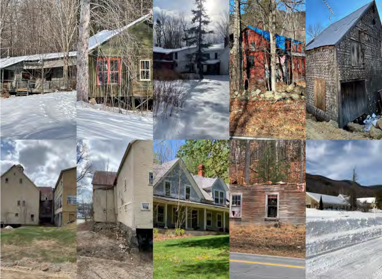
Various buildings in Jackson that were demolished
