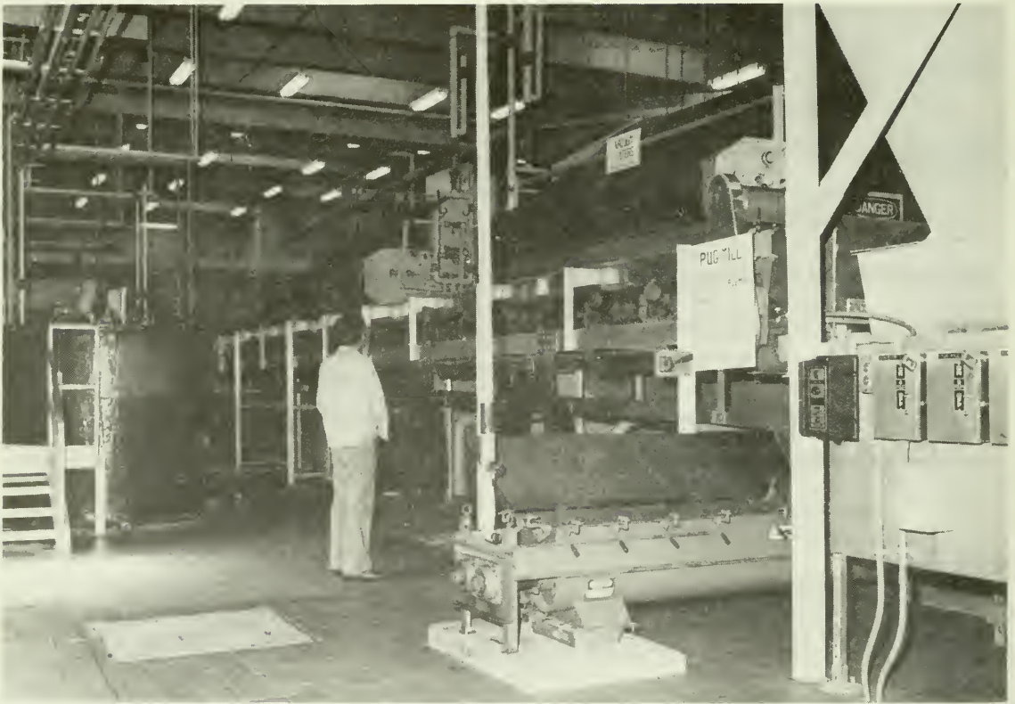
Sludge Processing and Wood Chip Mixing at the New Treatment Plant.
